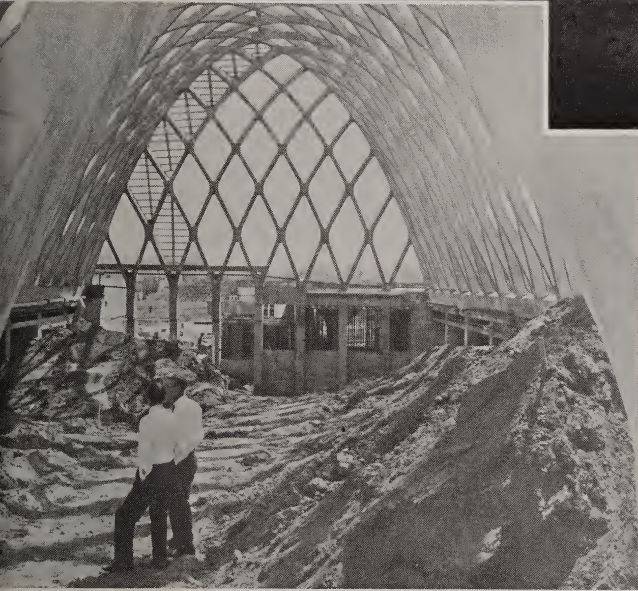
Looking East into the Unfinished Conservatory
