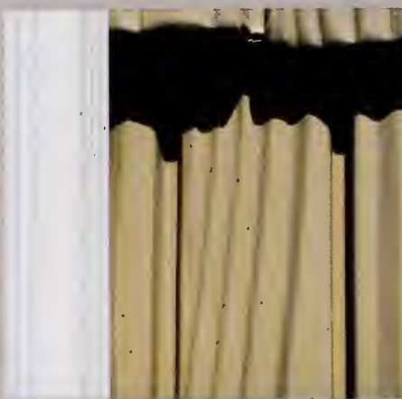
Artillery fungus (black spots) massed on the side of a house. The downspout (white) and aluminum siding (brown) are spattered with the black spots.
