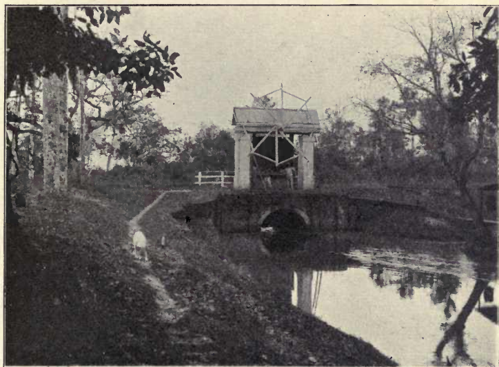
FIG. 129.—Sluice of the main drainage canal (plantation "Vredenburg").
