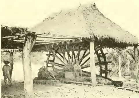
FIG. 85. Philippine sugar mill driven by water power
