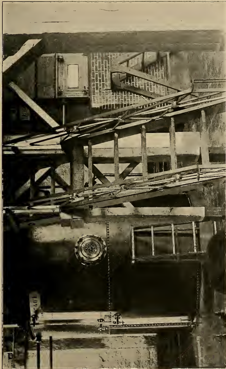
PLATE V. RECTIFYING APPARATUS AND BOILER IN PLANT OF AYALA AND COMPANY.
