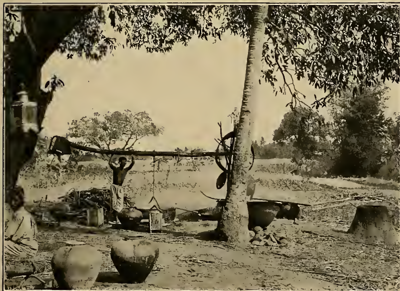
Fig. 2. Boiling works of basi mill.
