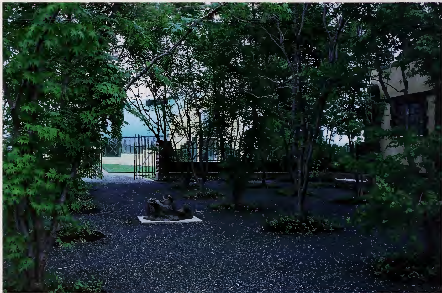
Top left: A stand of overgrown upright Japanese maples ( Acer palmatum ) are machine-dug at an abandoned nursery for the new courtyard. Top right: Asymmetrical trunks of Japanese maples are being precisely planted to contrast with the architect's symmetrical grid pattern. Bottom: The leafy canopy of the transplanted maples grace the new courtyard, sheltering a bronze sculpture by St. Claire Cemin.
