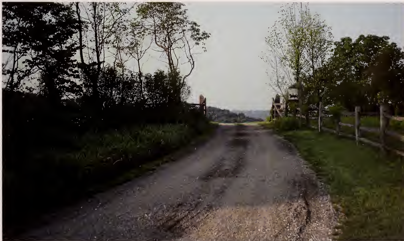
A hedgerow constructed from plants taken from abandoned fields, undeveloped lots or land soon to be developed, gives an immediate look of maturity and permanence and will continue to fill in as time passes.
