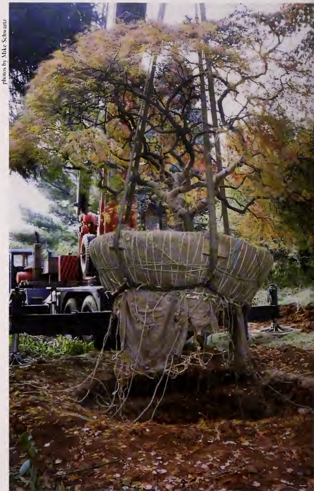
A 50-ton crane hoists a Japanese cutleaf maple ( Acer palmatum 'Dissectum') so that the bottom lacing can be tied to the ball before moving the tree to a new site. Over 100 pounds of twine and burlap were used.
