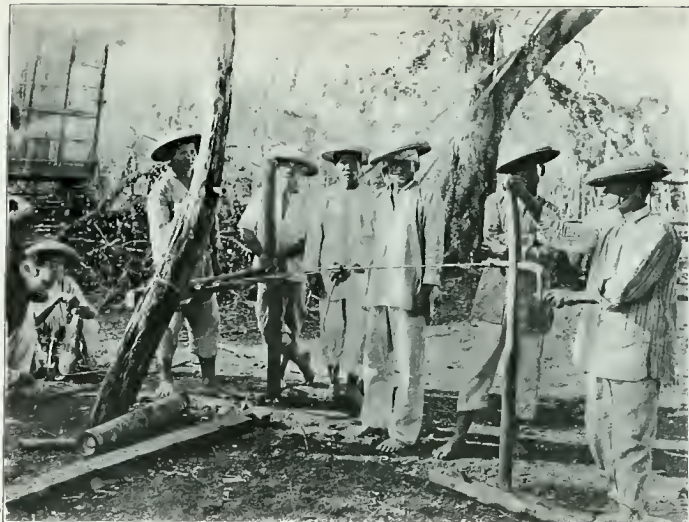
Fig. 1. Laying a three-strand rope.
