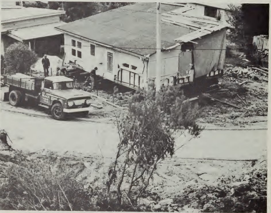
Plate 1. The house moved 5 m by the slip, so that it contacted the next house. The slip material has been removed.
